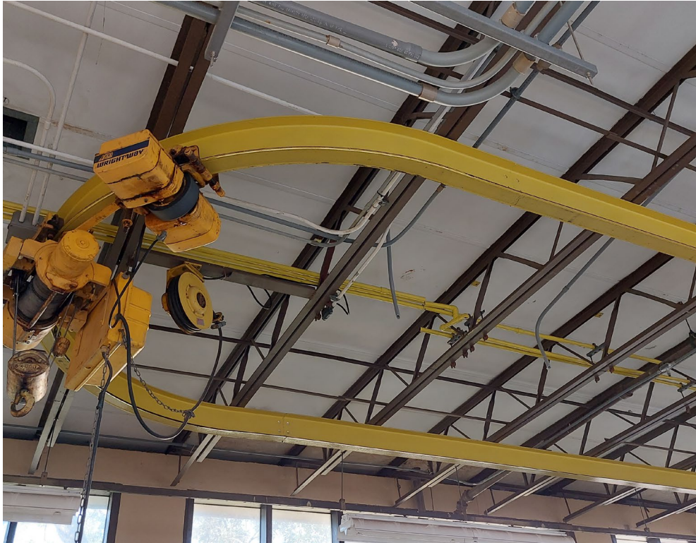
Photo 13 – LBP yellow metal crane/hoist inside Structure 12
