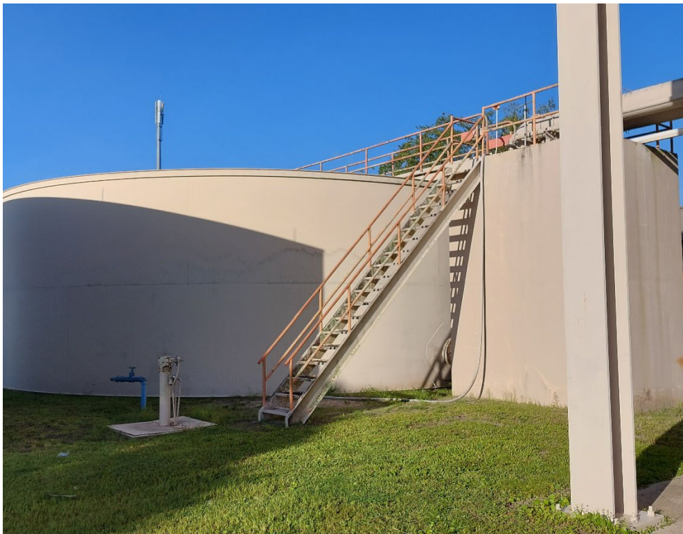
Photo 14 – LBP orange handrails on top of Structures 13 & 14
