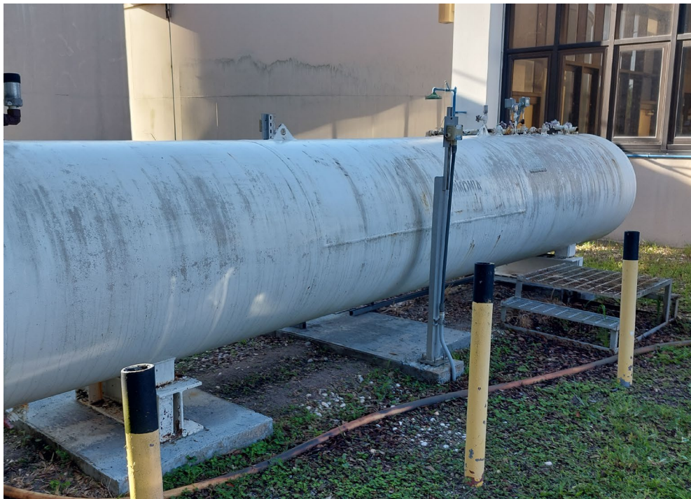
Photo 12 – LBP yellow metal parking bollards around Structure 11
