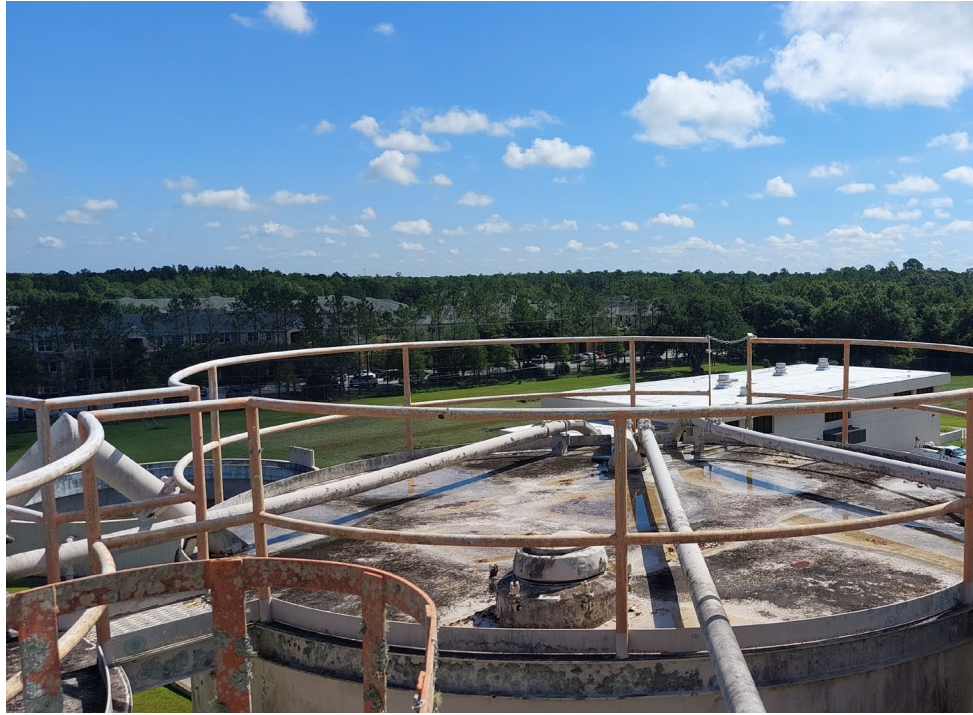
Photo 11 – LBP orange metal handrails on top of tanks/silos of Structure 10
