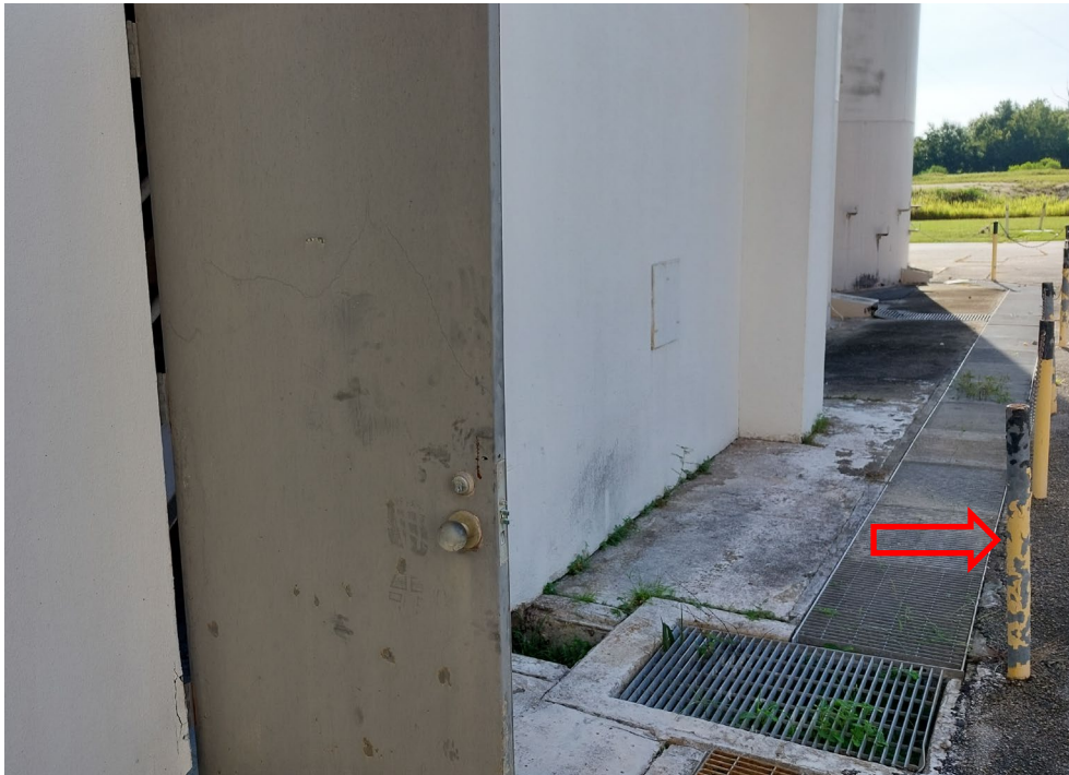
Photo 8 – Yellow metal parking bollards of Structure 9
