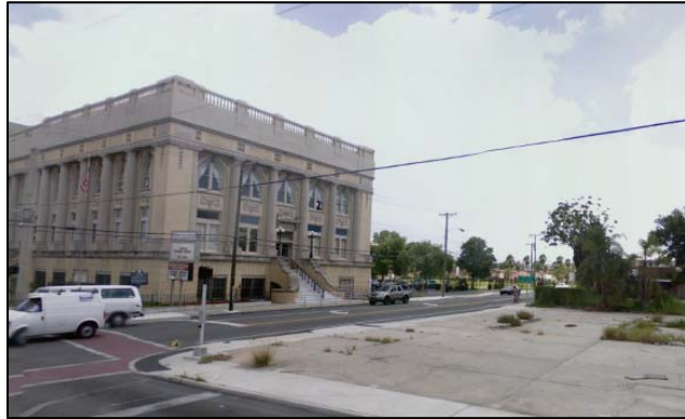
Redevelopment on vacant lots must be guided in a manner that respects the heritage of the corridor. ( Centro Asturiano pictured )
