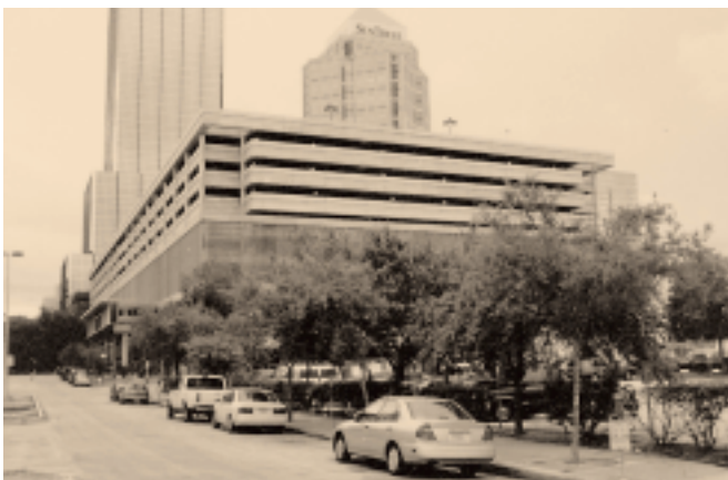
Fort Brooke Parking Garage expansion opened in July, 2000.
