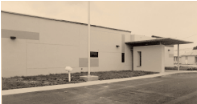
Fire and Police Communications Center
