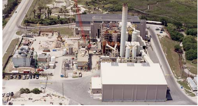
McKay Bay Refuse-to-Energy Plant Retrofit, scheduled for completion in early FY02.
