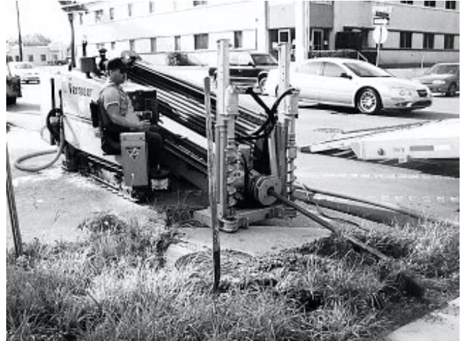
Directional Driller - saves digging up streets
