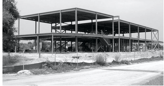
40th Street Maintenance Facility - open February, 2003
