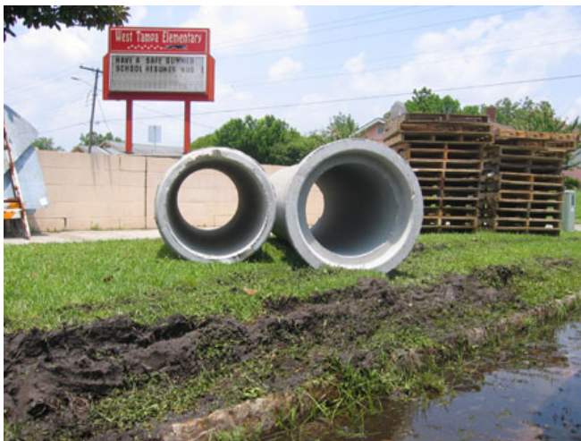
Stormwater project at West Tampa Elementary School.
