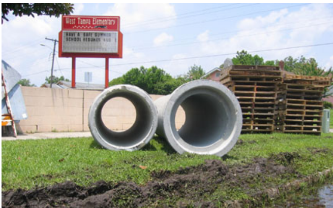
Stormwater project at West Tampa Elementary School.
