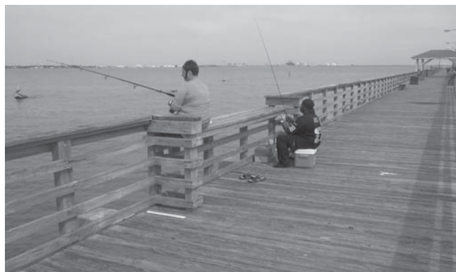
Ballast Point Pier
