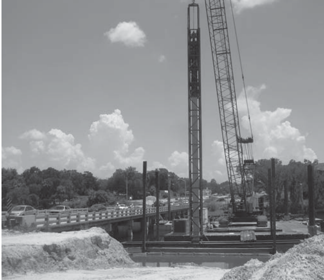
40th Street Bridge Construction
