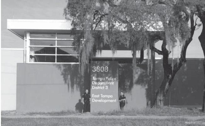
District III Police Headquarters
