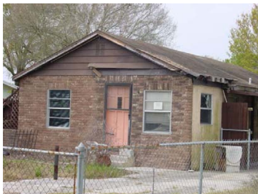
Before On-Site Replacement
