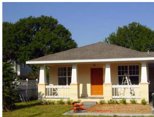
After On-Site Replacement
