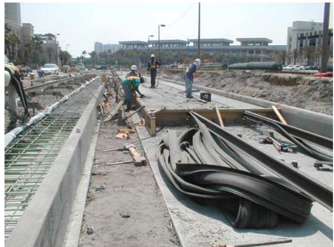
Streetcar construction on Ice Palace Drive.
