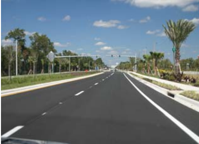
Completed Segment E
