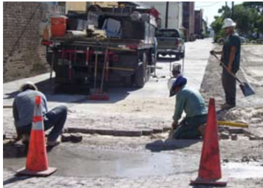
Brick apron under construction at the 1800 block of 7th Avenue.
