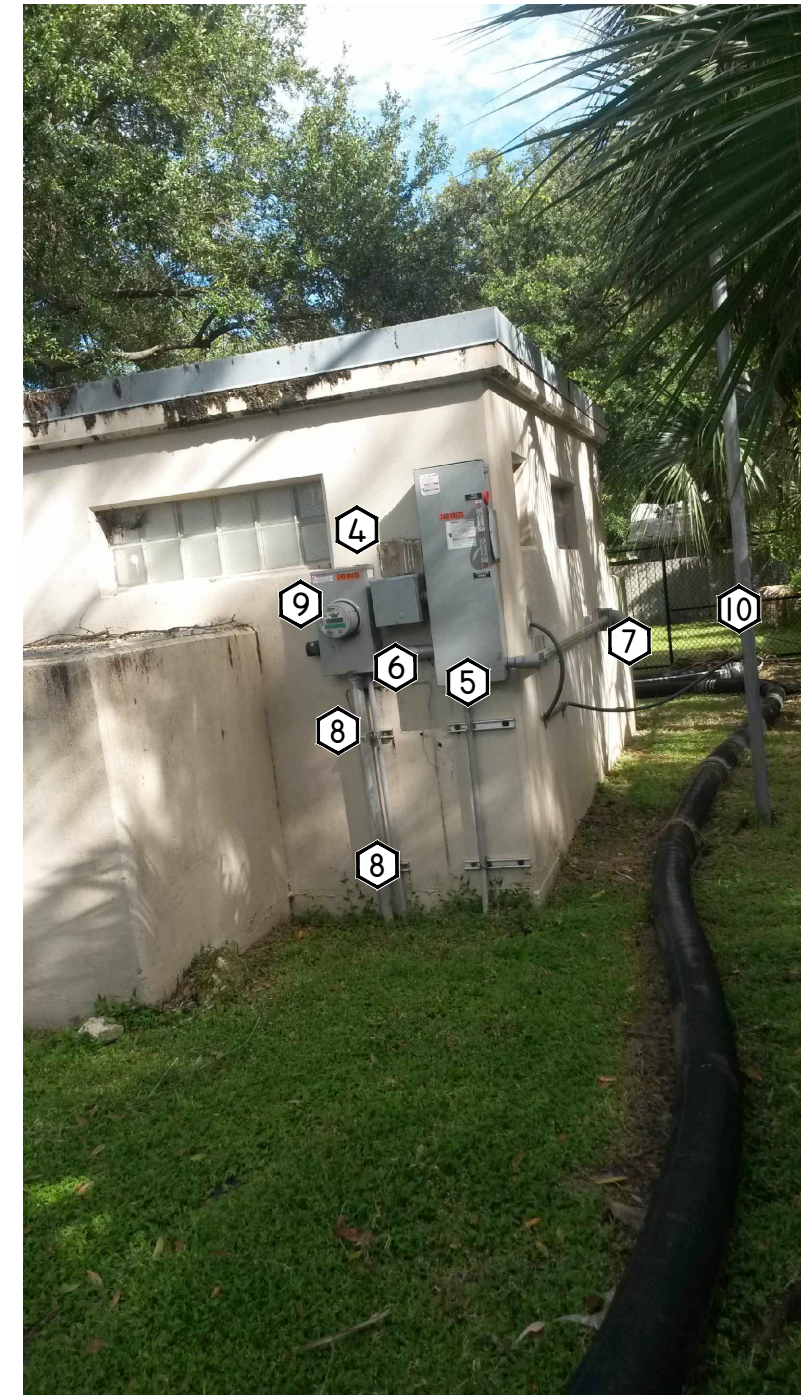
LOOKING NORTH, AT PUMPING STATION FROM THE PROPERTY LINE
