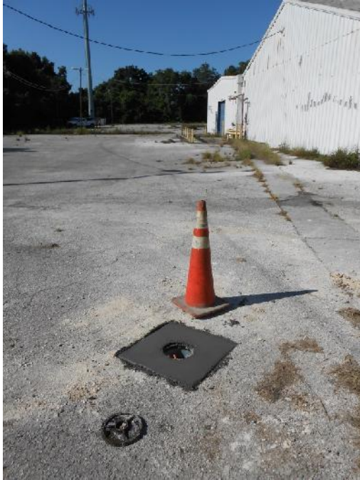
DW-1 Well Pad – Completed
