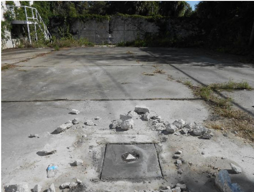
MW-7 Well Pad – Completed
