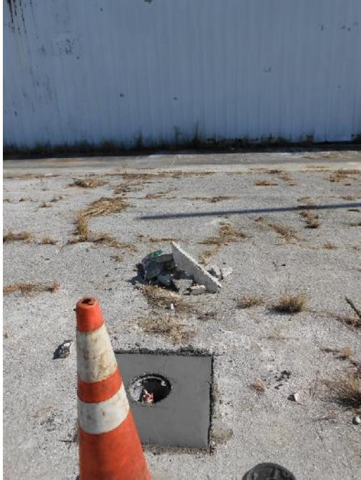
MW-6 Well Pad – Completed
