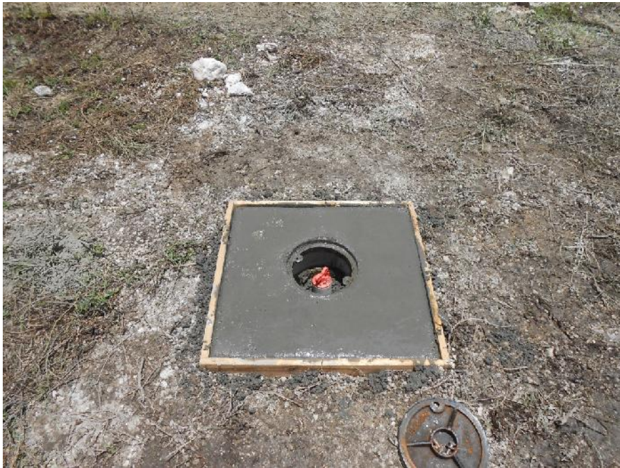
DW-2 Well Pad – Completed
