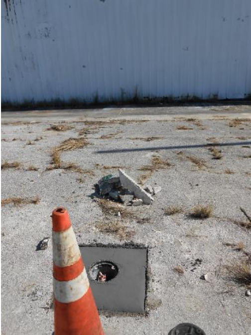
MW-6 Well Pad – Completed
