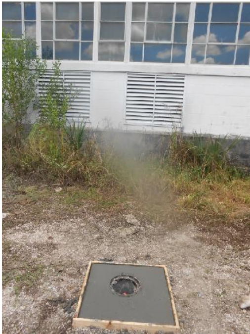
SW-1 Well Pad – Completed
