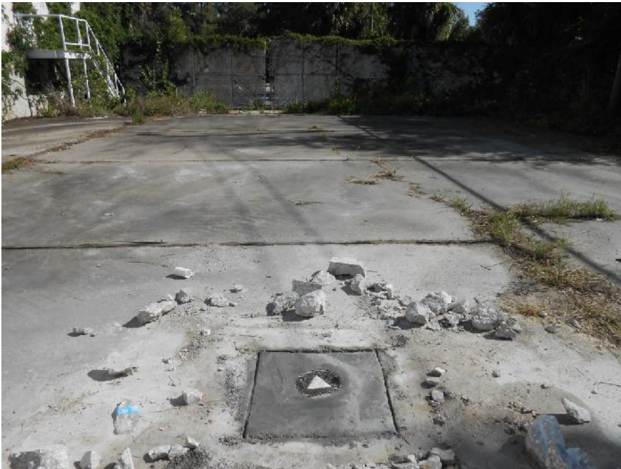
MW-7 Well Pad – Completed
