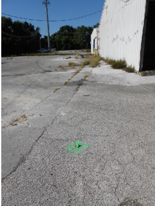
MW-4 – Completed by Others
