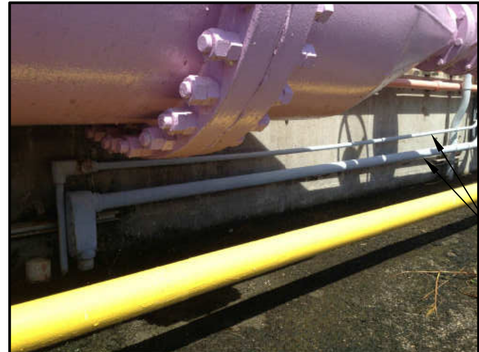
CONTRACTOR SHALL RELOCATE CONDUITS FOR THE INSTALLATION OF PROPOSED PIPE SUPPORTS
