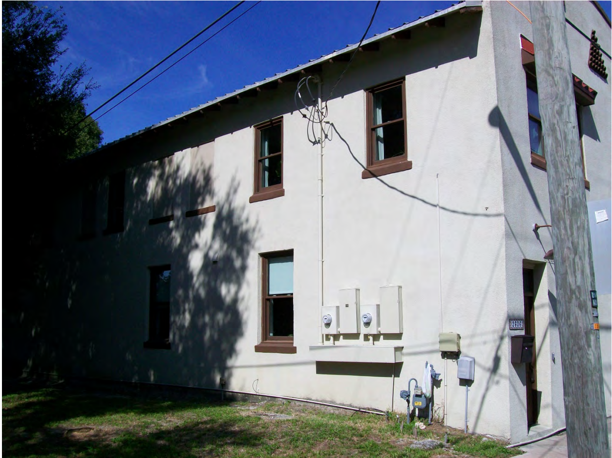
South Side of Building
