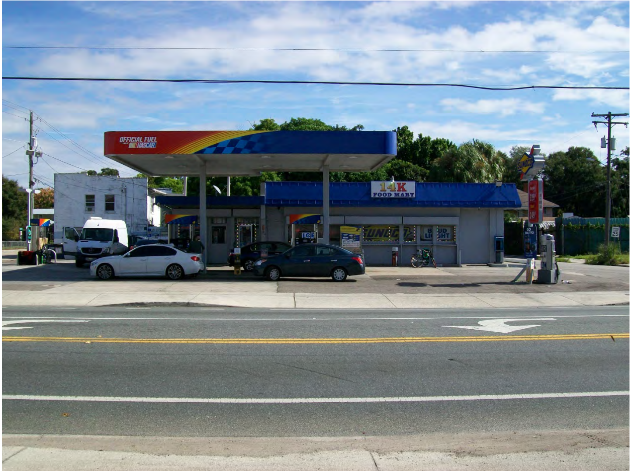
West Side of Building
