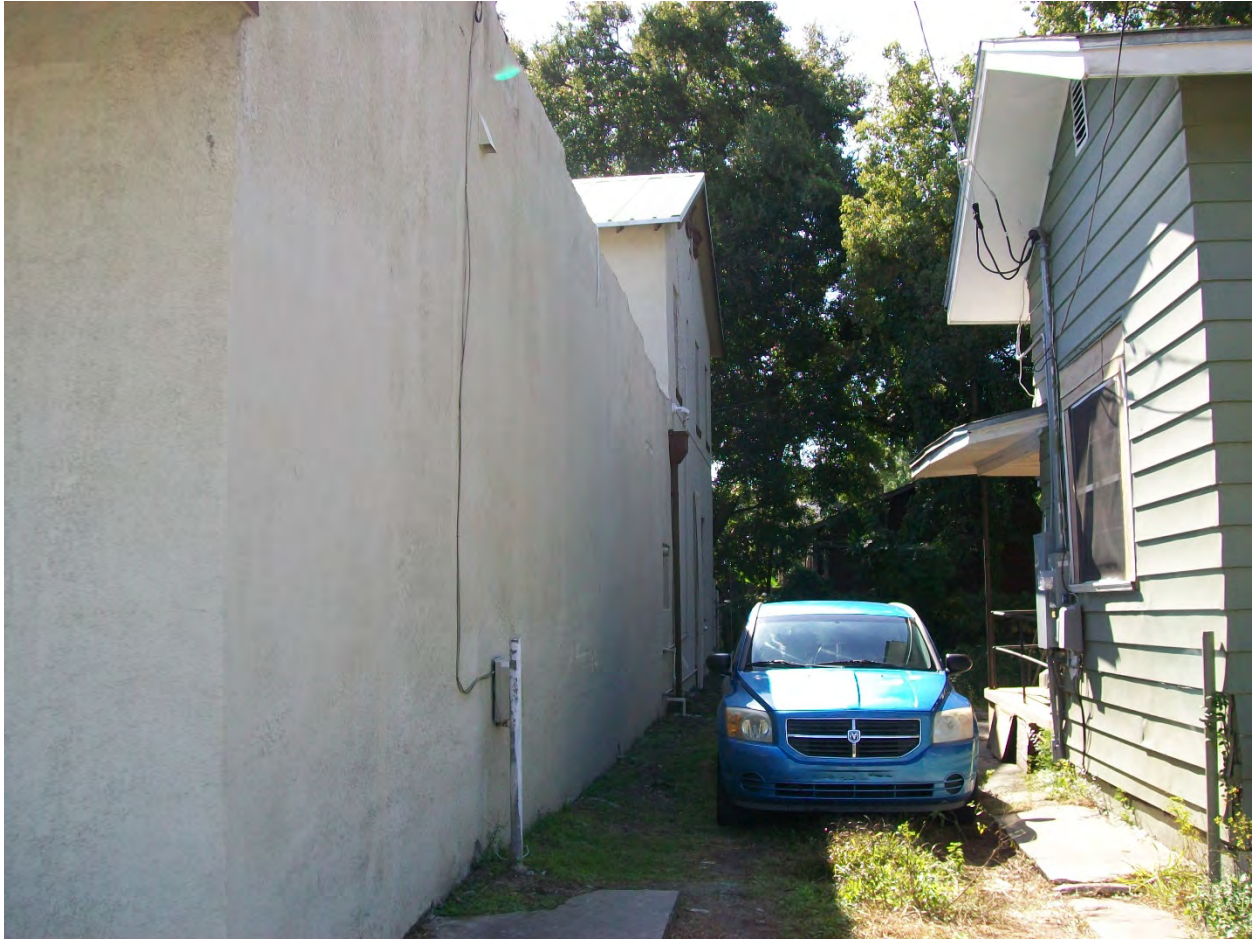
West Side of Building
