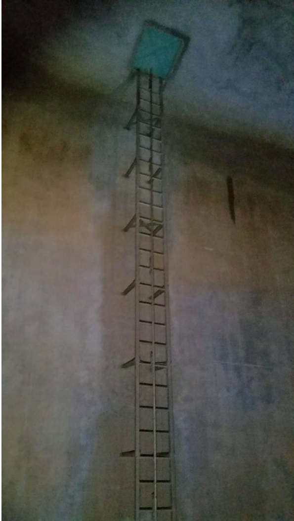
Figure 9 and Figure 10. MBPS East GST Interior Access Ladder Issues were not seen on the existing access ladder.
