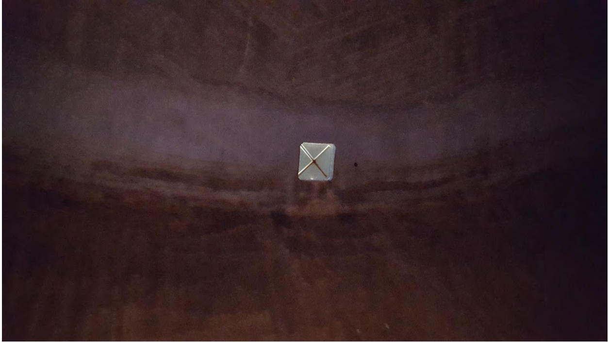
Figure 5. NWPS GST Hatch No access ladder from dome hatch.
