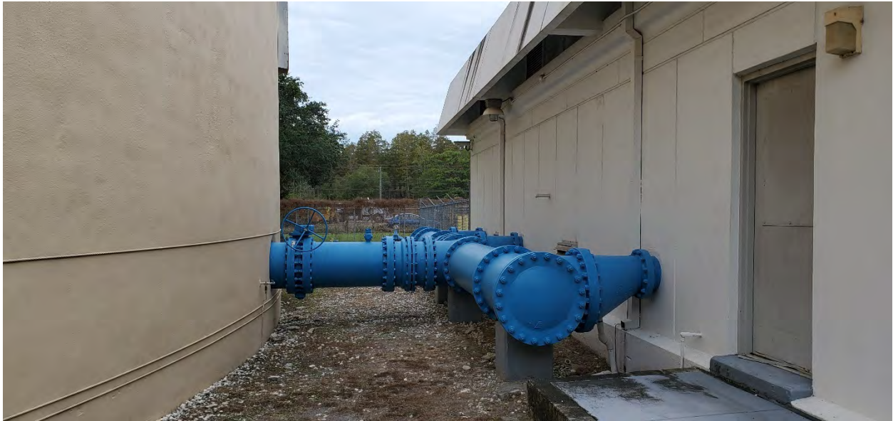
Figure 14. NWPS Building Exterior
