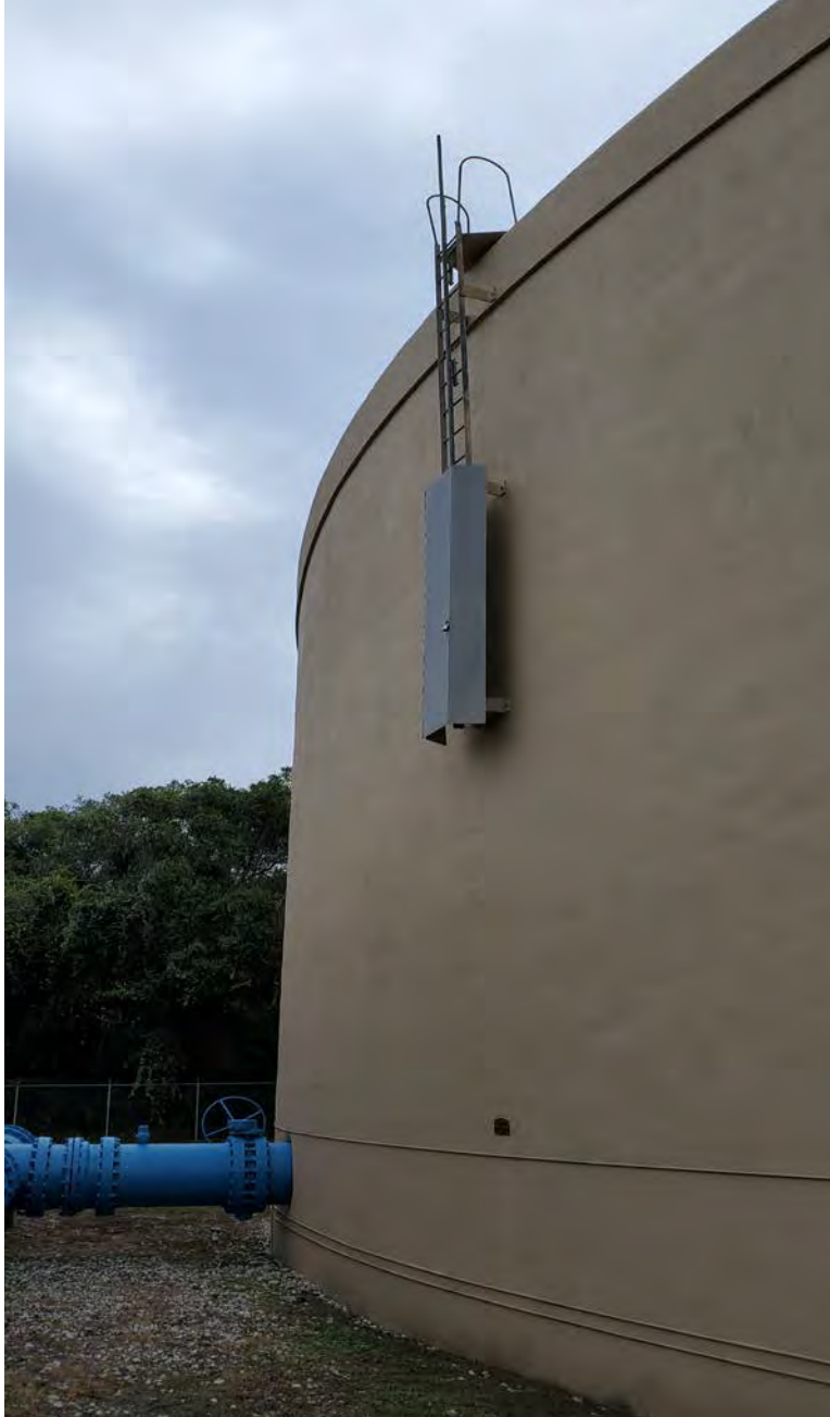
Figure 8. NWPS GST Exterior Ladder
