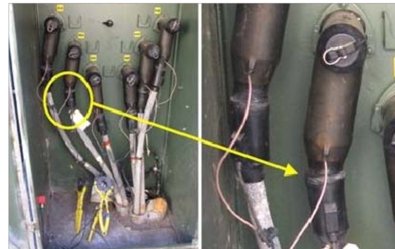
H2A BUSHING SHOWING DEFORMATION
