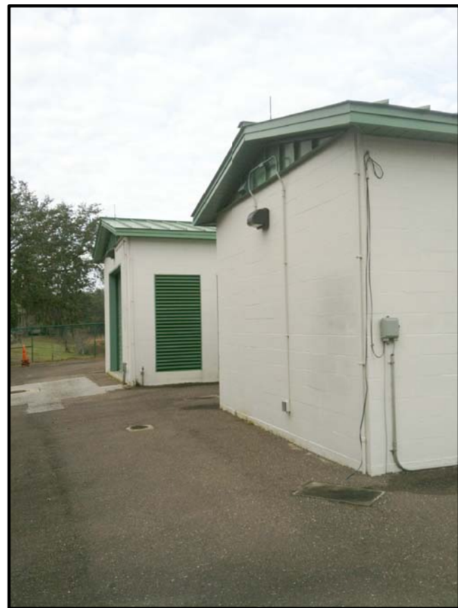
CURIOSITY CREEK STORMWATER PUMP STATION
