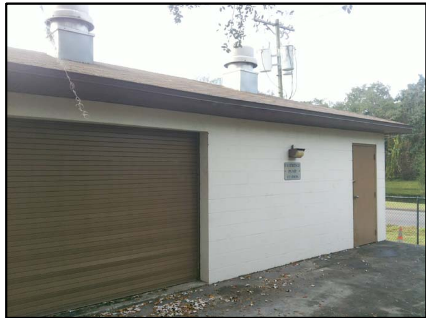
EASTRIDGE STORMWATER PUMP STATION
