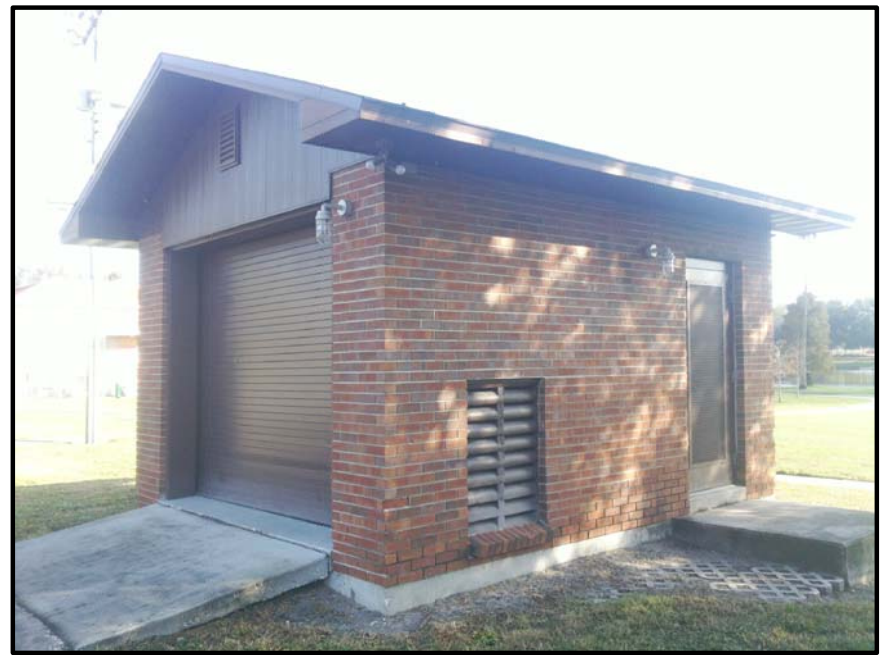
ROBLES PARK STORMWATER PUMP STATION
