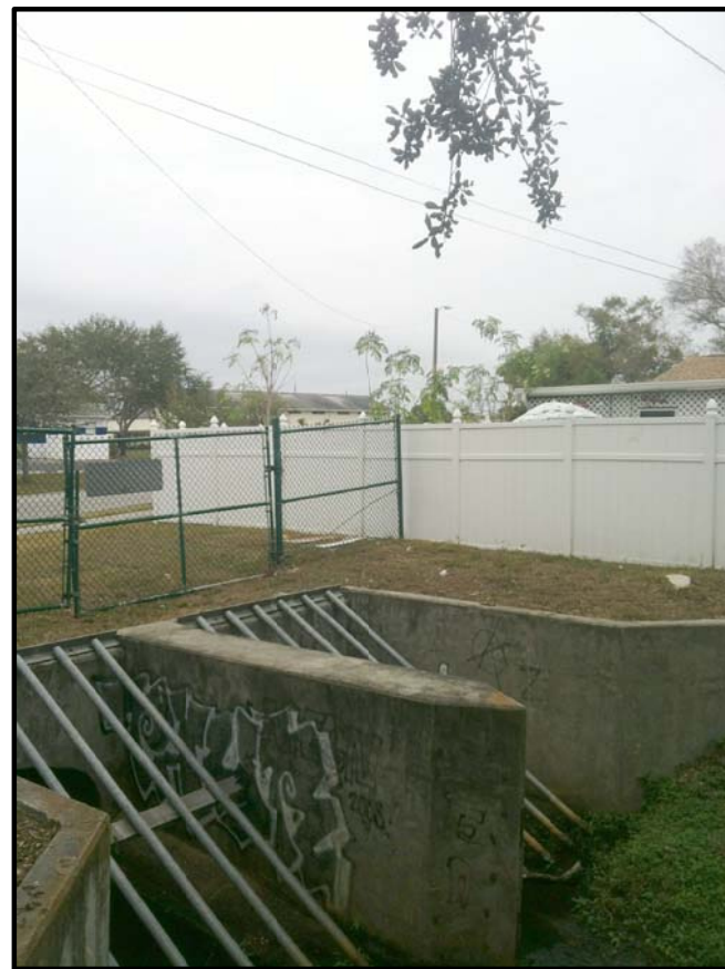
COOLIDGE GRATE DITCH
