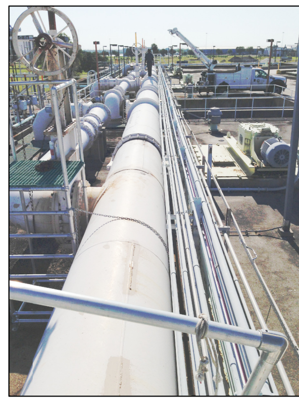
EAST VIEW FROM PLATFORM
