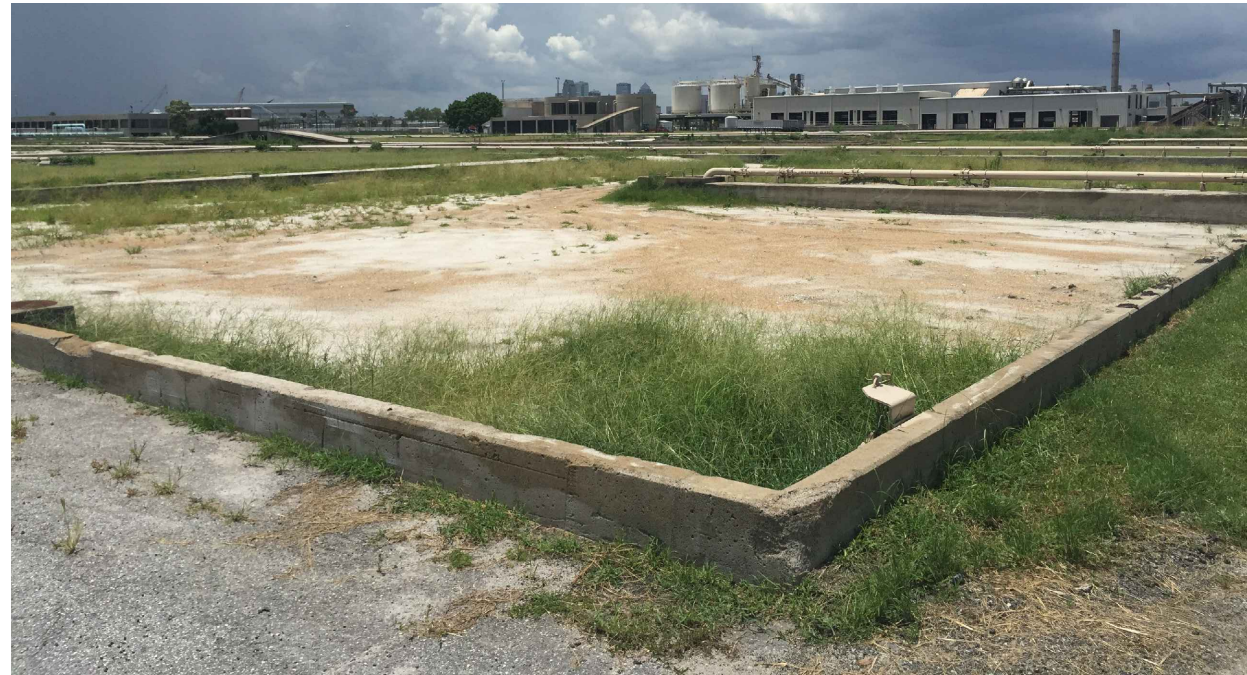
SLUDGE BED 32 (SOUTHEAST CORNER LOOKING NORTHWEST)
