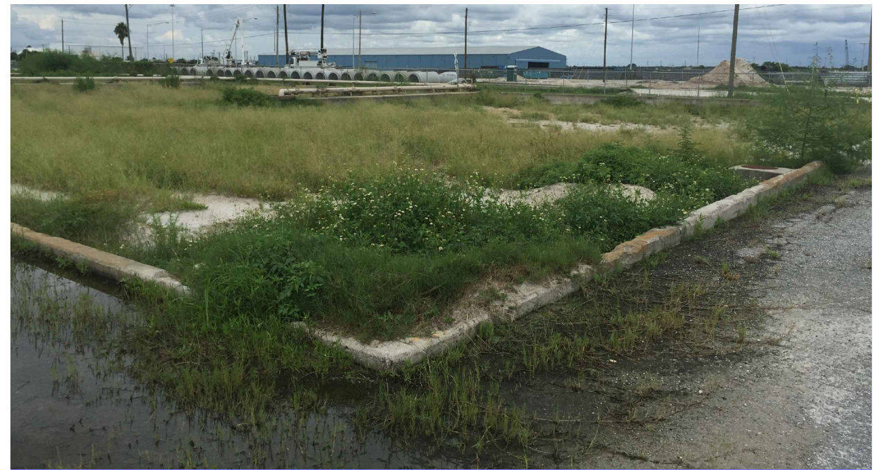
SLUDGE BED 32 (SOUTHWEST CORNER LOOKING NORTHEAST)
