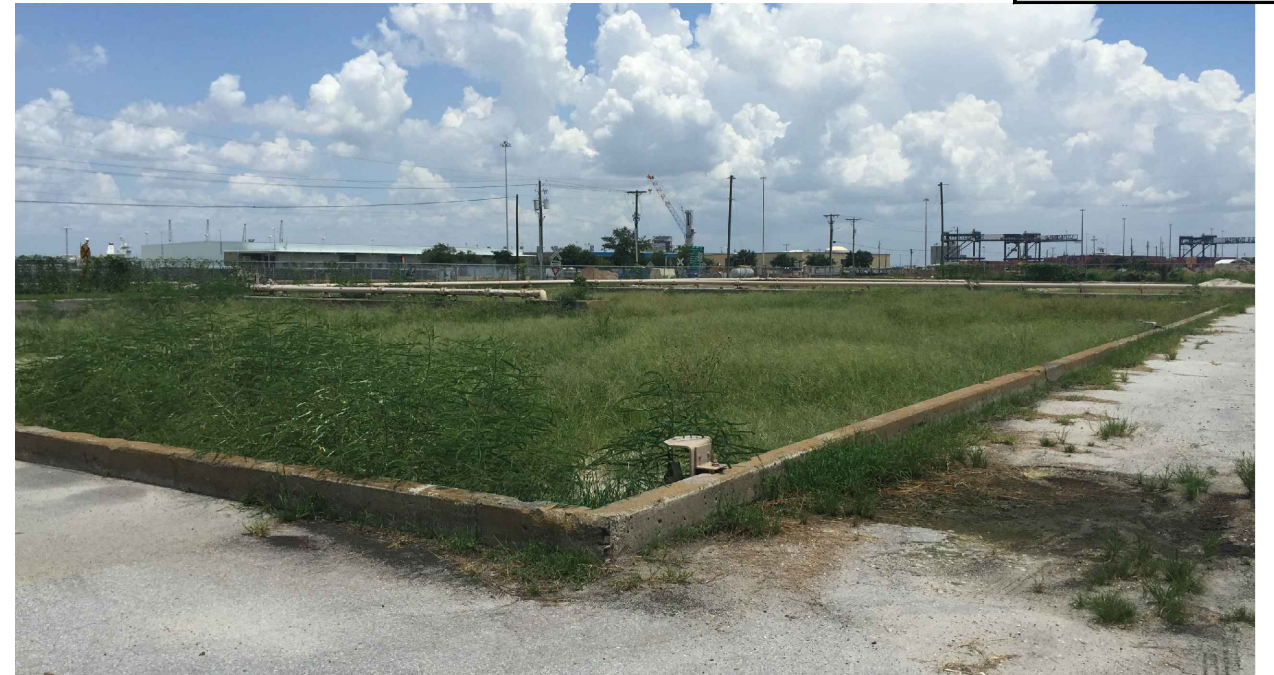
SLUDGE BED 24 (NORTHWEST CORNER LOOKING SOUTHEAST)
