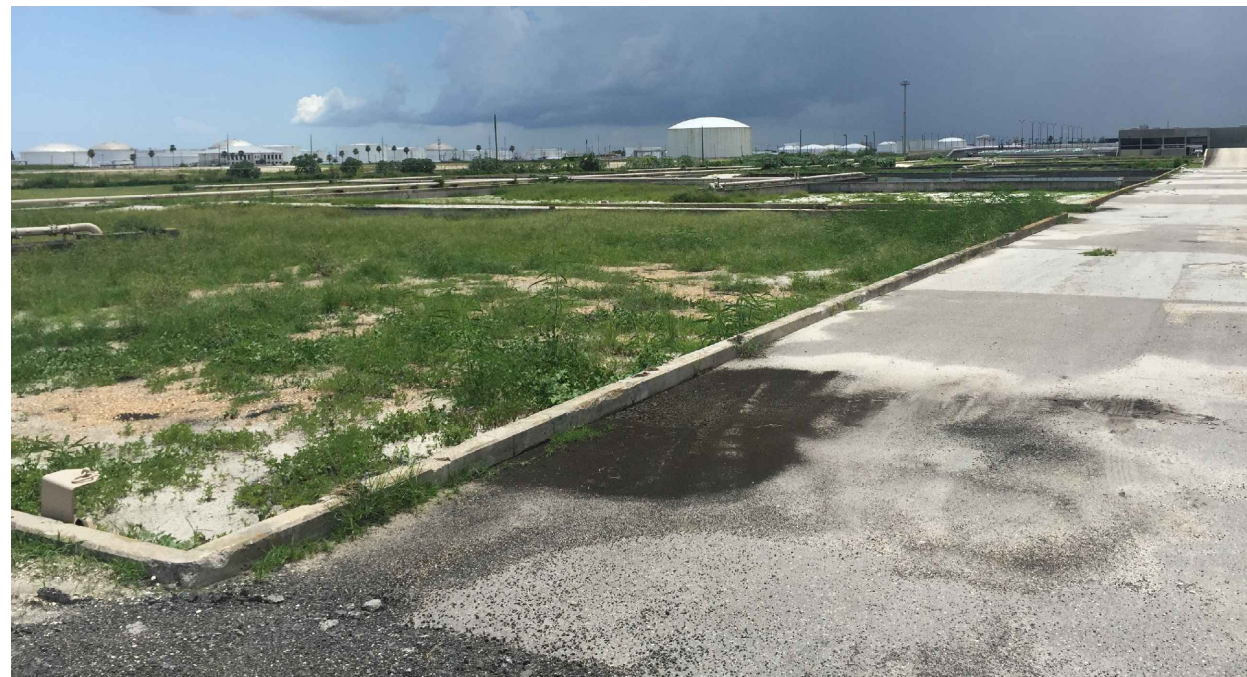
SLUDGE BED 24 (NORTHEAST CORNER LOOKING SOUTHWEST)
