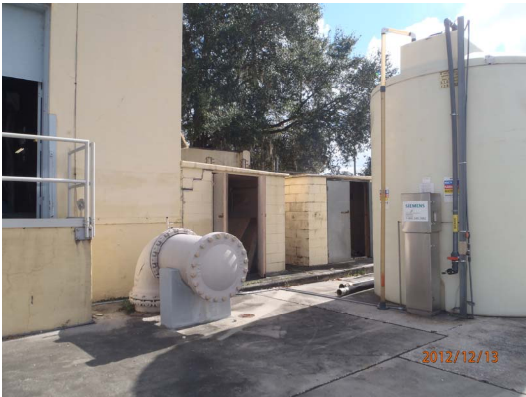
Photograph 4- General view of small sheds behind building
