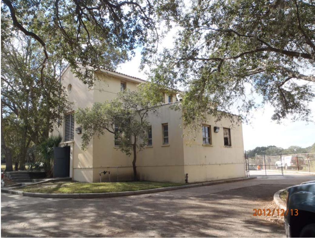
Photograph 1- General view of the building,
