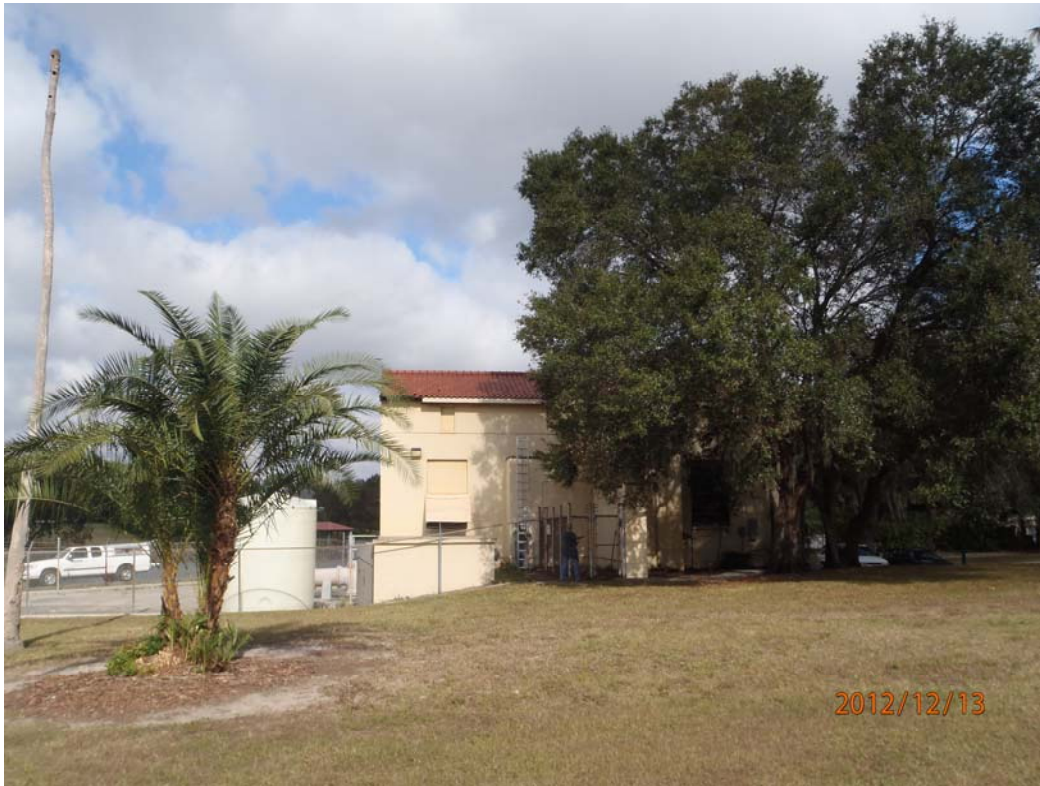
Photograph 5- General view of south side of building.
