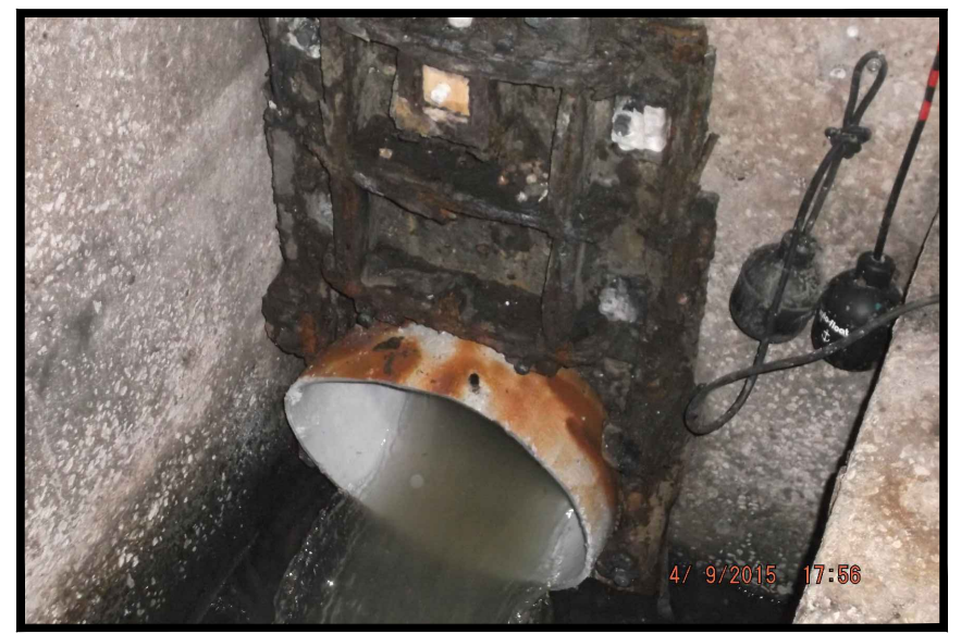
* PHOTO OF EX. LINER THROUGH EX. SLUICE GATE NOT TO SCALE
