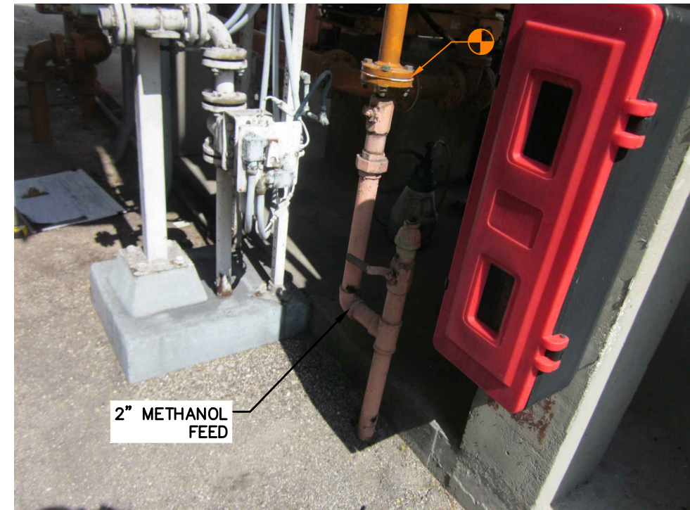
METHANOL FEED PIPING REMOVAL LIMIT
