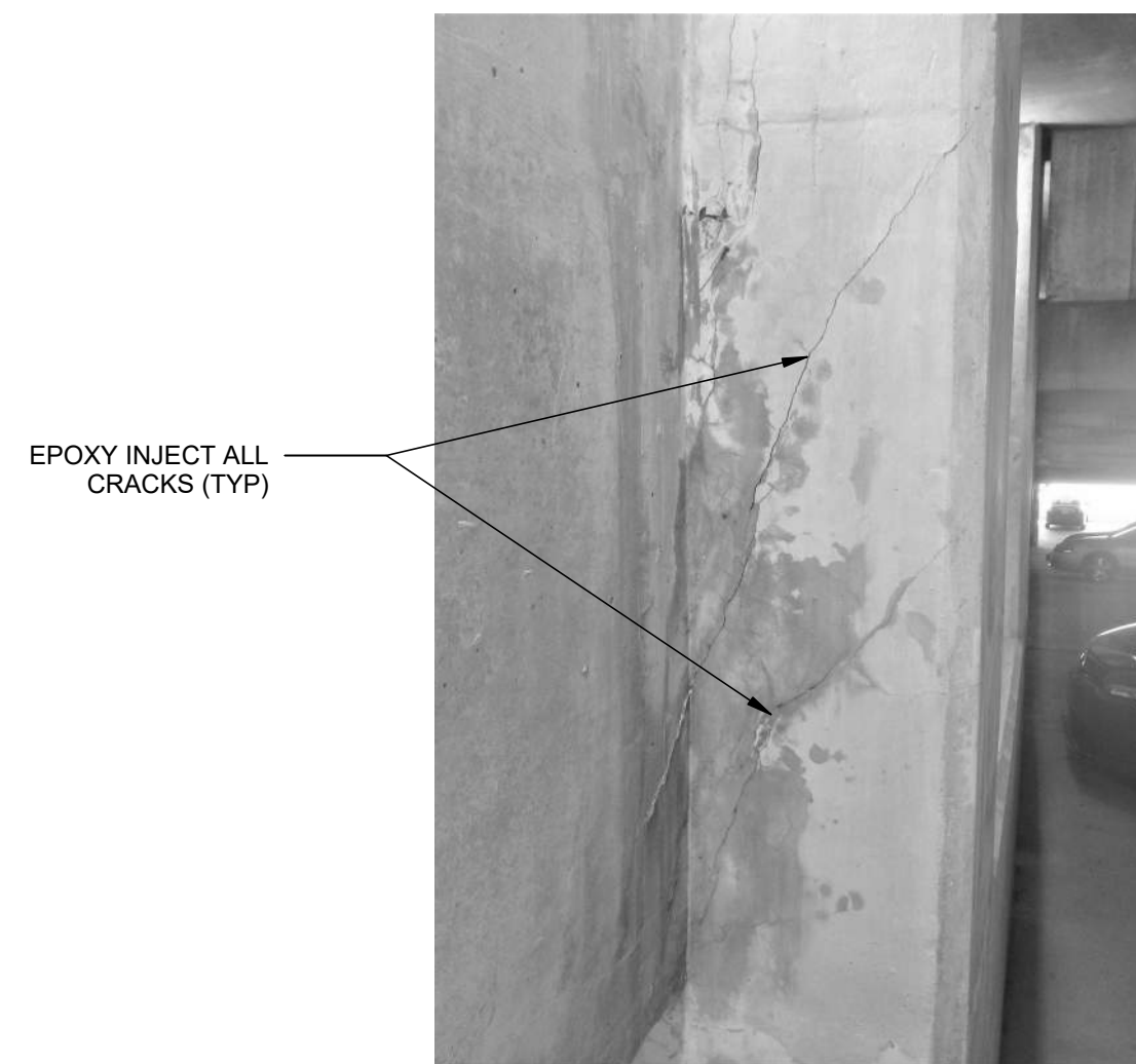
TYPICAL EXISTING CONDITION AT COLUMN
