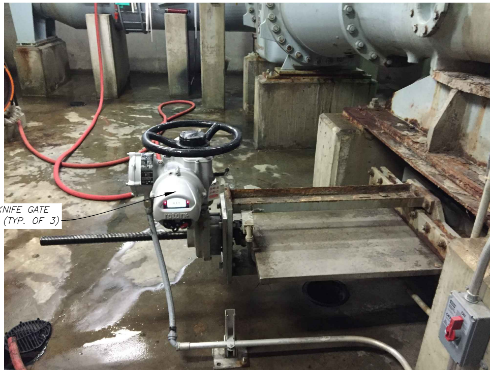
PROPOSED CONFIGURATION FOR KNIFE GATE VALVE ACTUATORS
