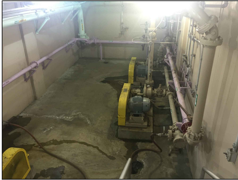
EXISTING CONDITIONS - NORTH - 1 - KING - T
