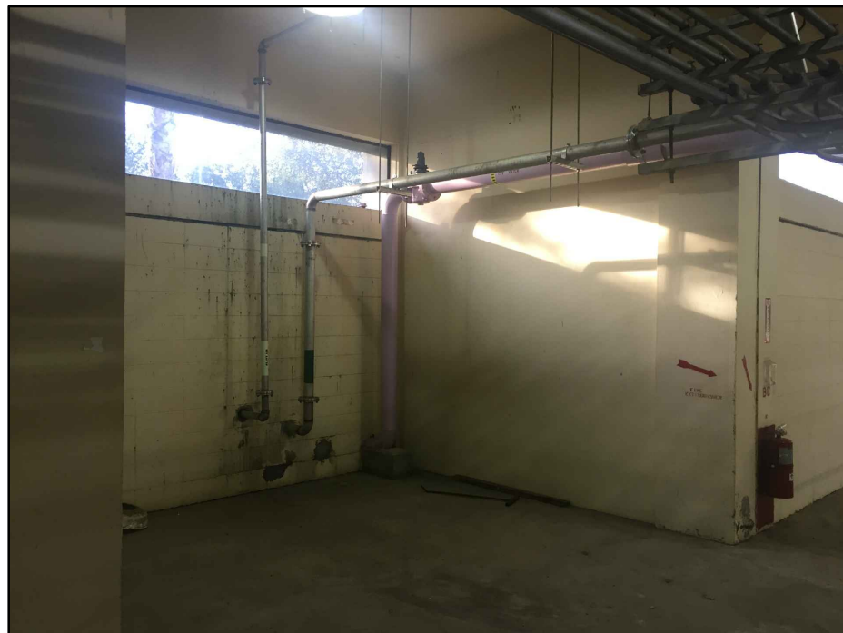
EXISTING CONDITIONS - LOOKING NORTHWEST
