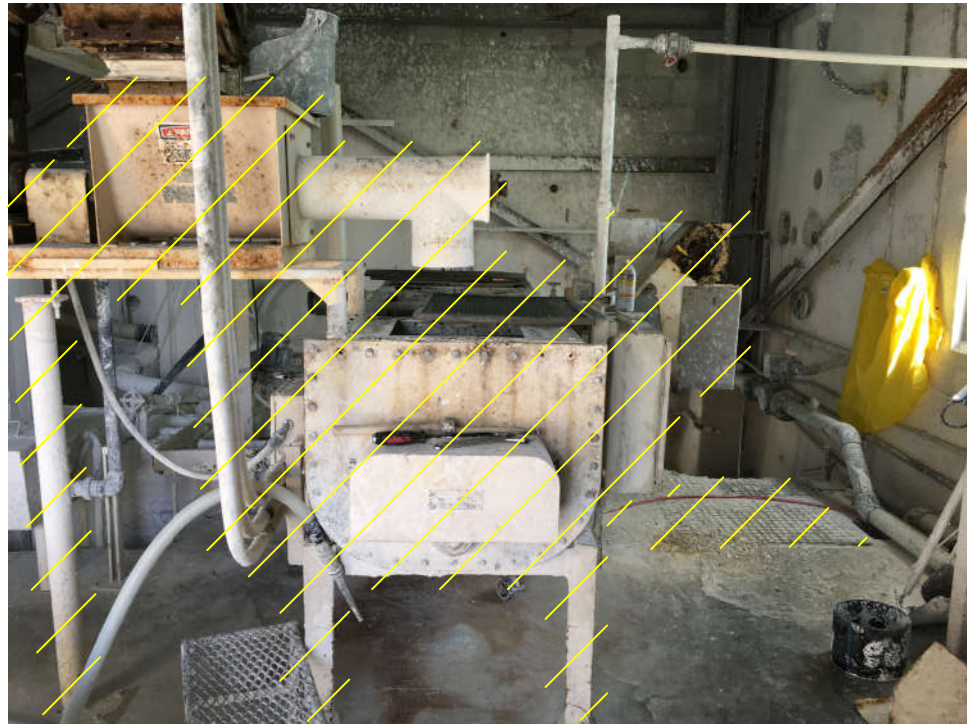
DEMOLITION OF EXISTING OLD SLAKER – VIEW 1
