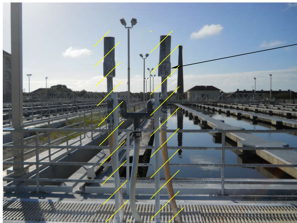
DEMOLITION OF EXISTING LIME DOSING ASSEMBLY
