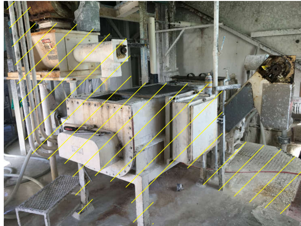
DEMOLITION OF EXISTING OLD SLAKER – VIEW 2
