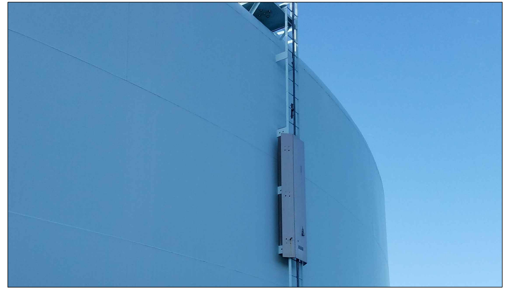
Figure 3 - Coat exterior ladder rungs with non-skid coating as specified.
