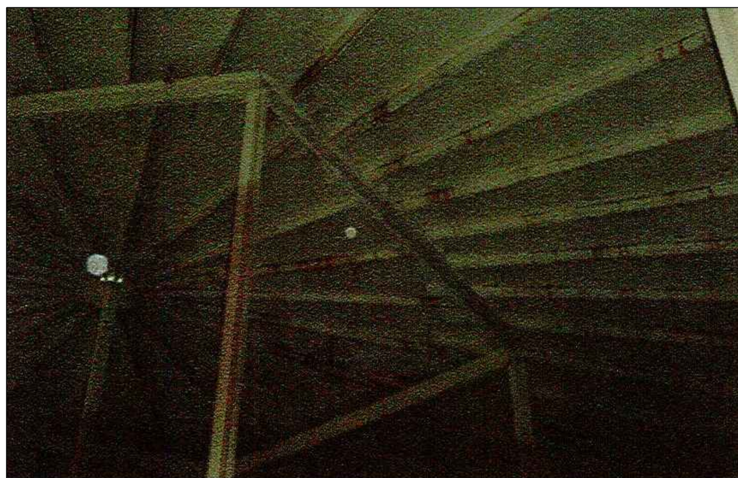
Figure 7 - All rafter surfaces exhibiting rust shall be cleaned and re-coated as specified.
