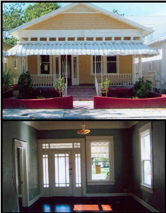
Residential Structure “After”
