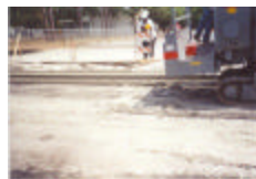
WMBE's perform all types of work. This is E/S Concrete.
