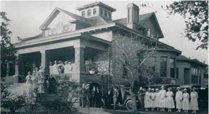
Group portrait of staff in front of Bayside Hospital on Bayshore Boulevard in 1920. Built by Tampa City Council member Silas Leland Bigelow in 1908, the house was sold to Dr. John Sullivan Helms in 1917, and became Bayside Hospital, the first private hospital on the west coast of Florida. It closed in 1927, when Tampa General Hospital opened on Davis Islands. The house still stands today on Bayshore Boulevard.
