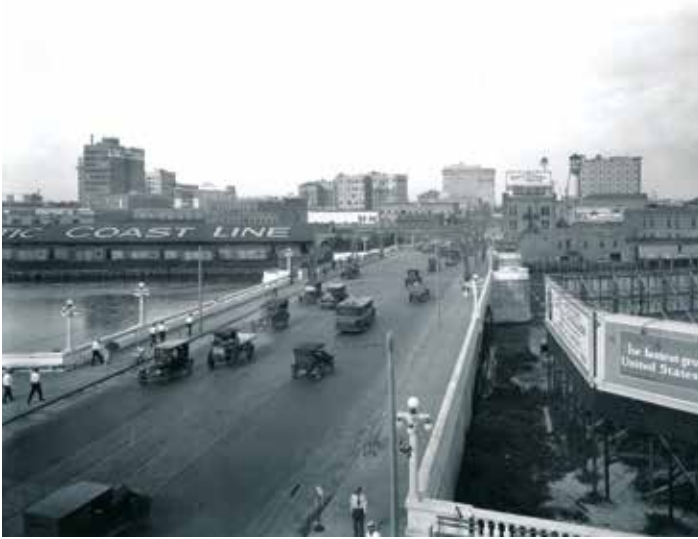
The Lafayette Street Bridge looking east toward downtown in 1920.
