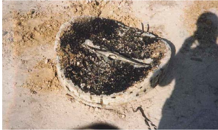
Photograph 9 – 36-inch Coupon, June 22, 1987, Convention Center Pipeline Relocations
