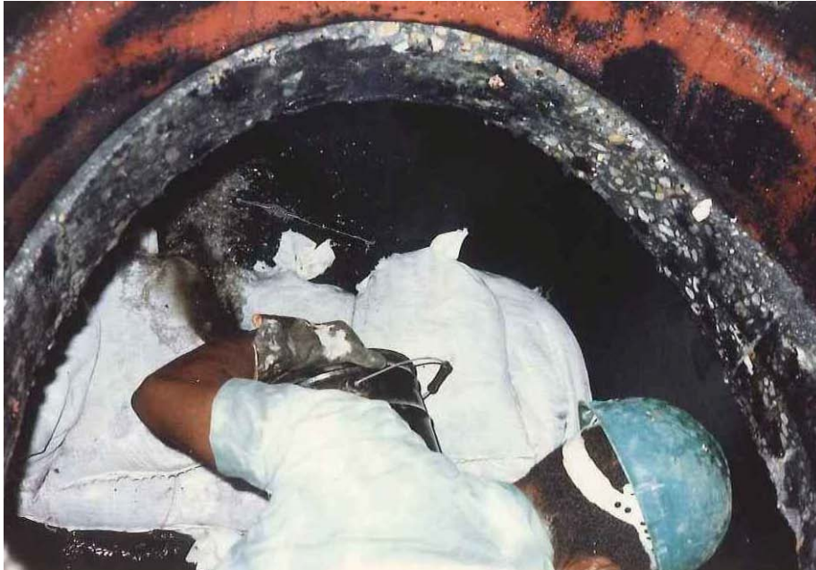
Photograph 7 – Cut Pipe Wall, June 26, 1987, Convention Center Pipeline Relocations
