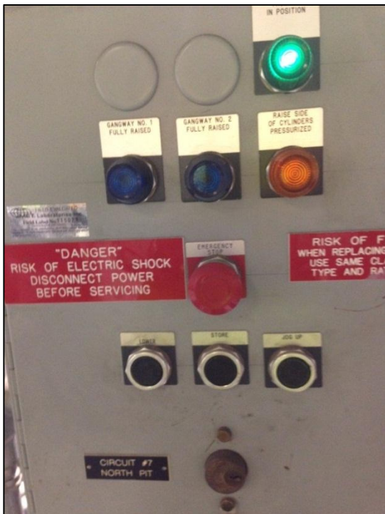
PHOTO 11 INTERLOCK PANEL
