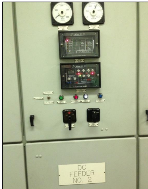
PHOTO 15 PROTECTIVE RELAYS
