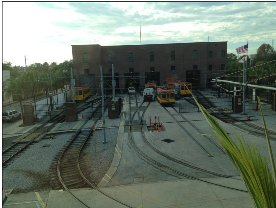
PHOTO 10 VIEW OF VMF YARD TRACKS
