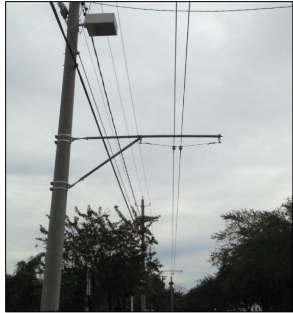
PHOTO 23 CANTILEVER ARM BOWING
