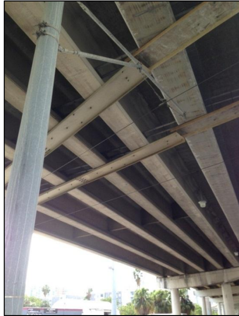
PHOTO 28 OCS POLE UNDERNEATH BRIDGE
