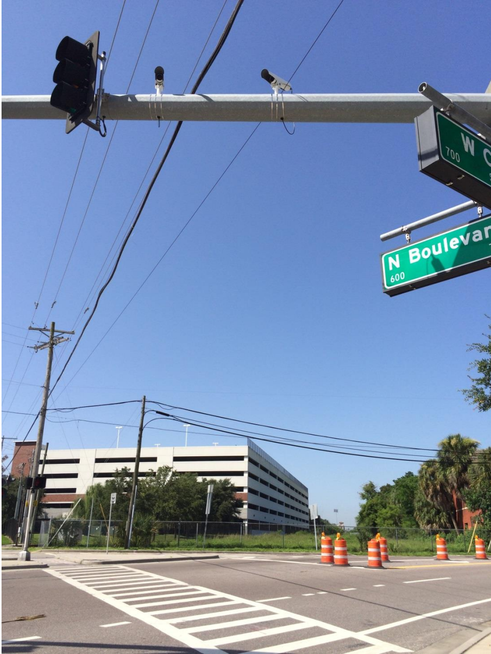
Intersection of N Boulevard and Cass Street (downstream portion of project), looking SW
