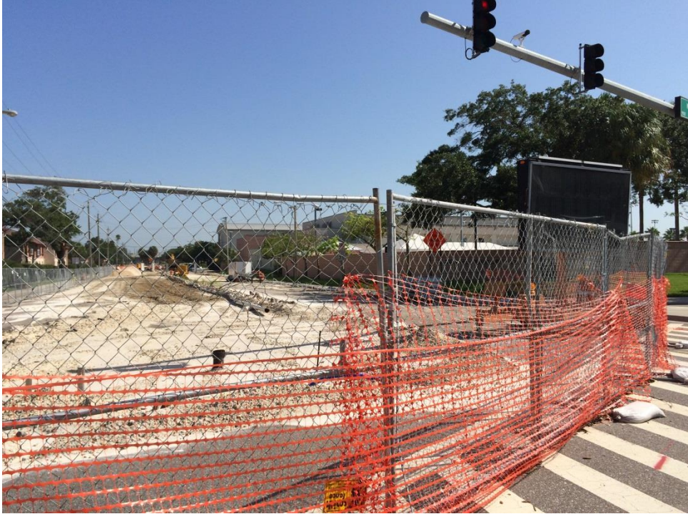
Construction along N Boulevard of twin 9' x 7' box culvert, looking N
