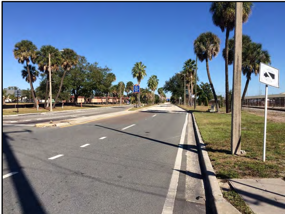
Looking east into the intersection of Nuccio Parkway and Nebraska Avenue
