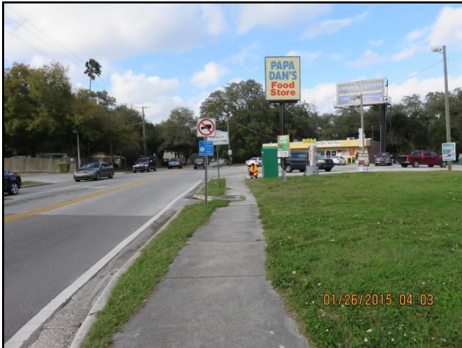
Looking north on the east side of 46 th Street. Begin project at Bush Blvd.
