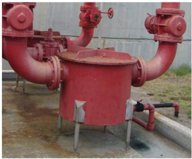
Figure 4-4: Biogas Condensate/Sediment Trap
