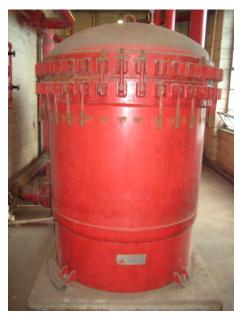
Figure 4-3 - Biogas Conditioning Filter
