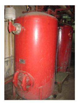
Figure 4-6: Pressurized Biogas Condensate/Sediment Trap
