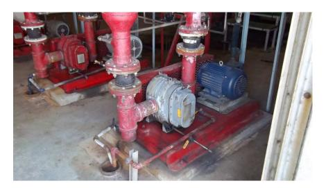
Figure 4-2: Biogas Compressors
