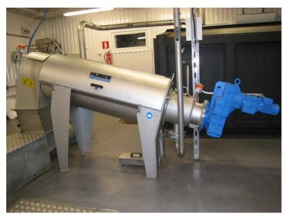
cleaned with spray water from the outside. The screw stops and reverses rotating the basket through 360° allowing the spray bar to fully wash the exterior surface of the basket within the enclosure. The screw pushes dewatered sludge to the upper end of the basket where it compressed against a pressure cone maximizing dewatering performance before discharging and dropping down a chute into a dumpster.
