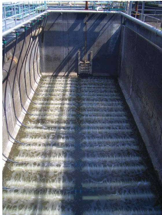
Figure 2. Two basic methods of in-basin piping. Left picture is conventional SS drop to PVC laterals (laterals may also be SS). Right picture is 2-inch HDPE drops connected to two to six individual diffusers. HDPE or flexible PVC 1-in tubing with compression fittings connects individual diffusers in both cases. More installation pictures are included in Attachment C.
