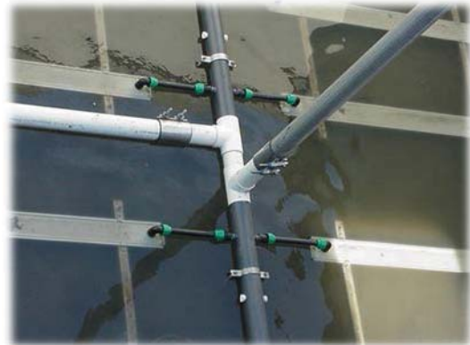
Connection "Q" Type to PVC Lateral Diffusers Mounted Above Sloped Floor
