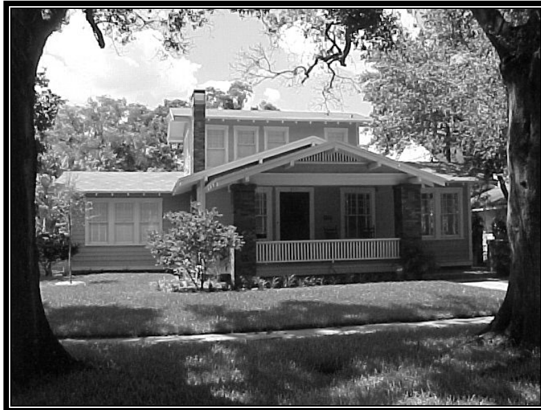
A one-story addition to the left of the original structure which is compatible with the existing.
